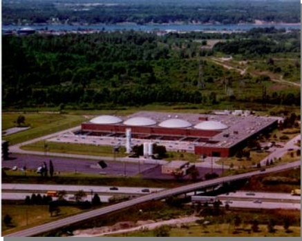
Tonawanda Wastewater Treatment Plant
