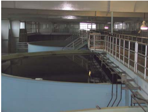
Keokuk Water Settling Tanks
