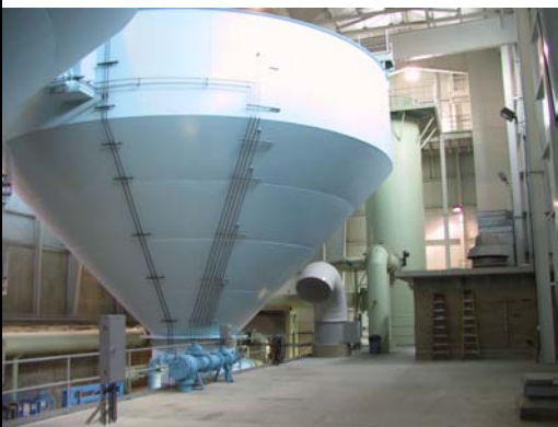
Keokuk Water Clarifiers
